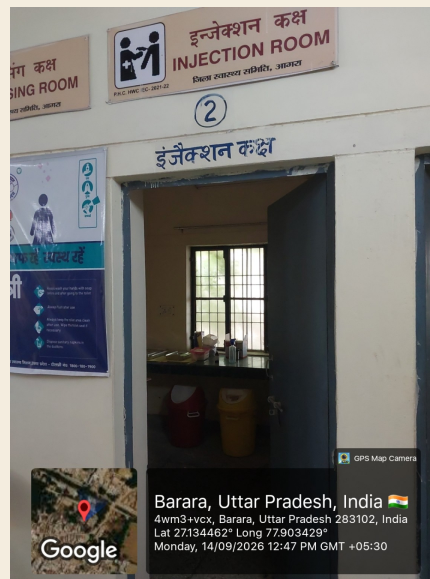
Injection room/service point at Barara.
