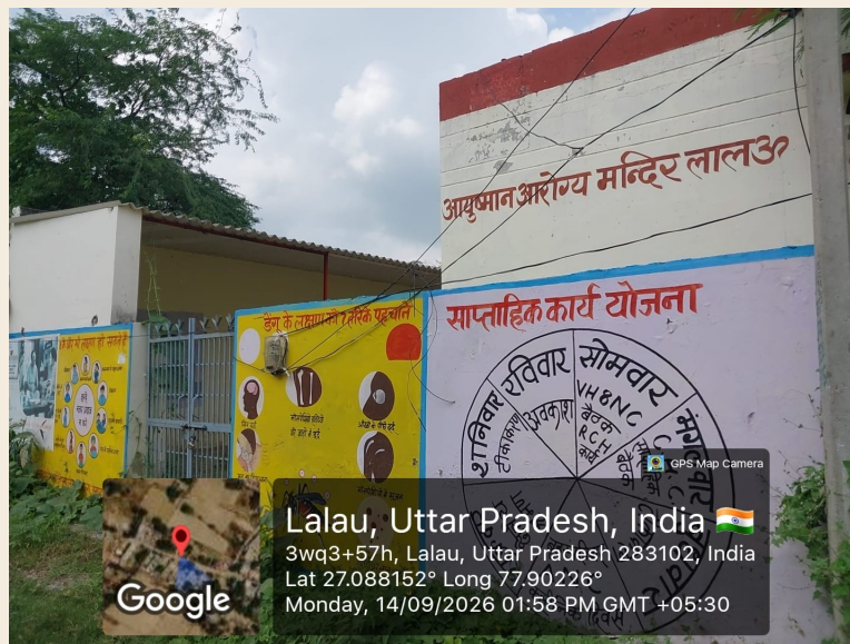
Additional exterior view of Lalau facility; internal access remained unavailable.
