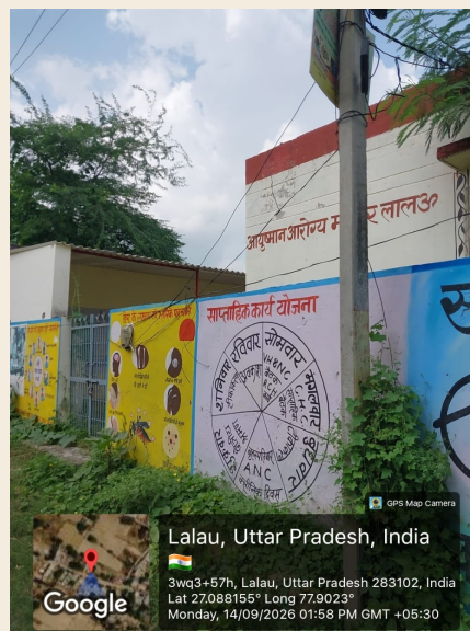
Front/exterior view documenting the facility from outside the locked premises.
