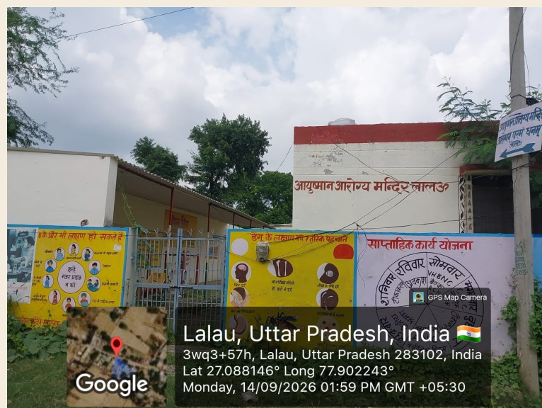
Exterior view of Lalau facility and public-health wall information.
